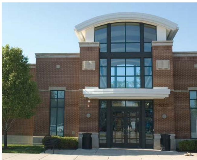
Chicago Public Library, West Pullman Branch
