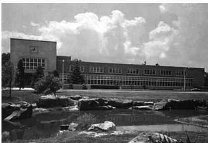
Early view of Morris Library, Southern Illinois University, Carbondale, currently under renovation and expansion
